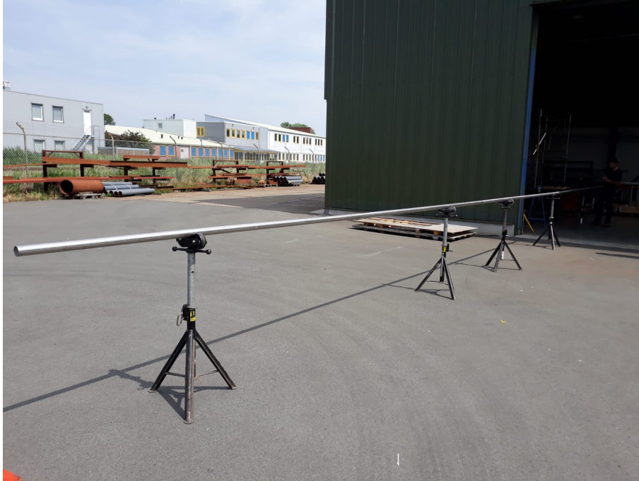
Figure 31: Main pipe at the factory.
