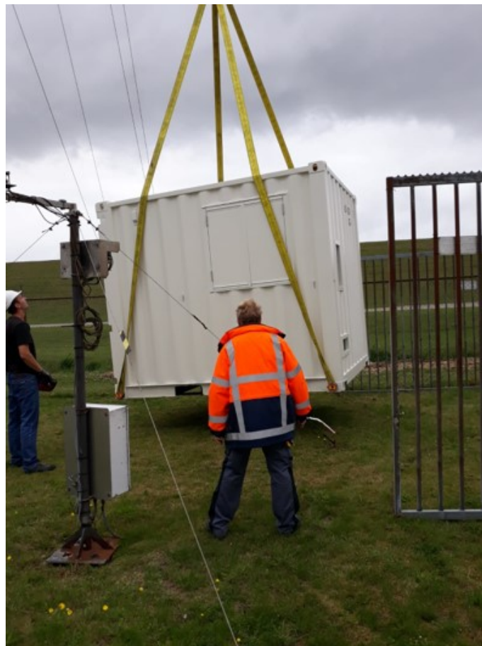
Figure 41: The placement of the container.
