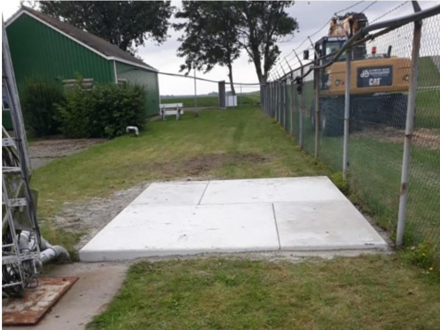
Figure 40: The foundation for the container next to the Lutjewad tower.
