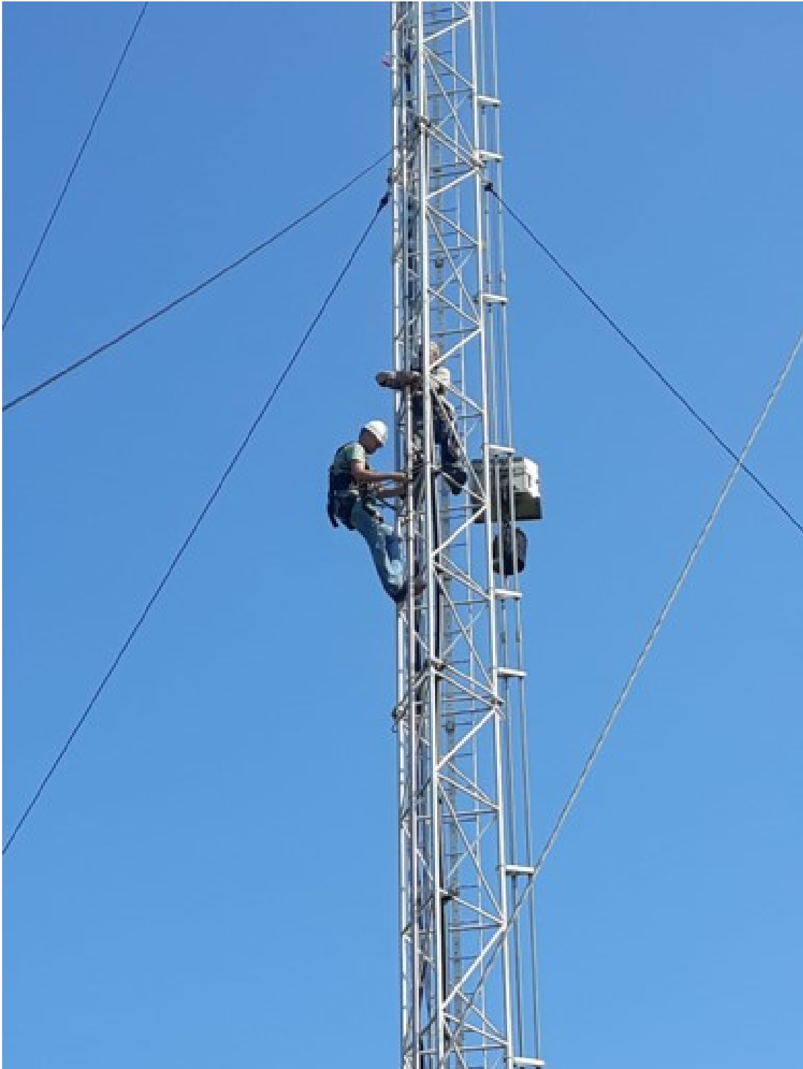
Figure 35: Attaching the main pipe to the Lutjewad tower.
