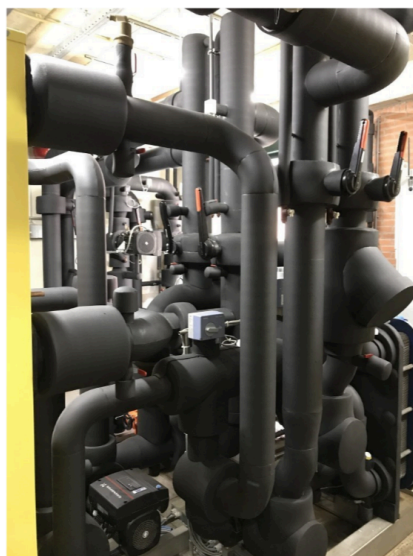
Figure 7: ATEs Pump for Underground Water Extraction
