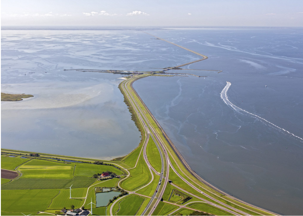
Figure 3.1: The Afsluitdijk, with the Wadden Sea on the right and the IJsselmeer on the left.
