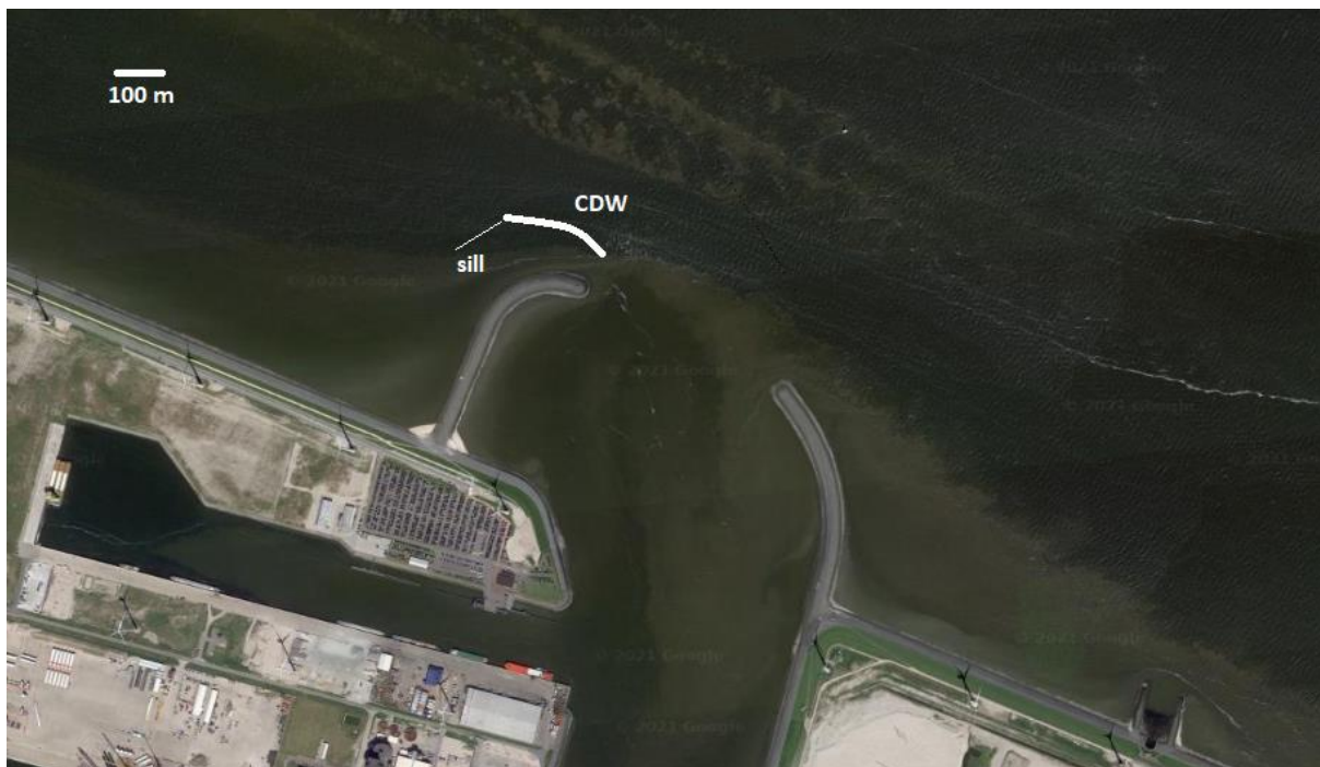
Figure 27: Rough sketch of the CDW and sill. Picture taken and adapted from Google Earth.
