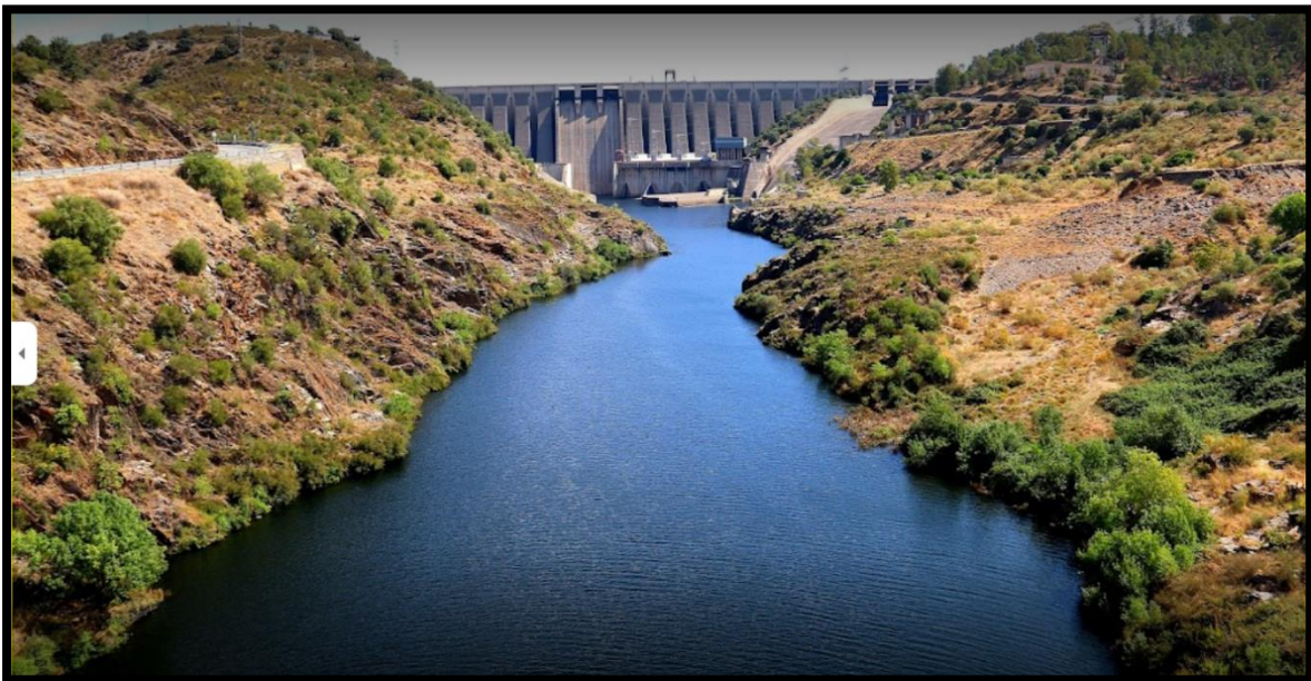
Figure 4: Alcantara Hydropower plant (J.M Oriol Hydropower plant)(Google Maps, n.d.)
