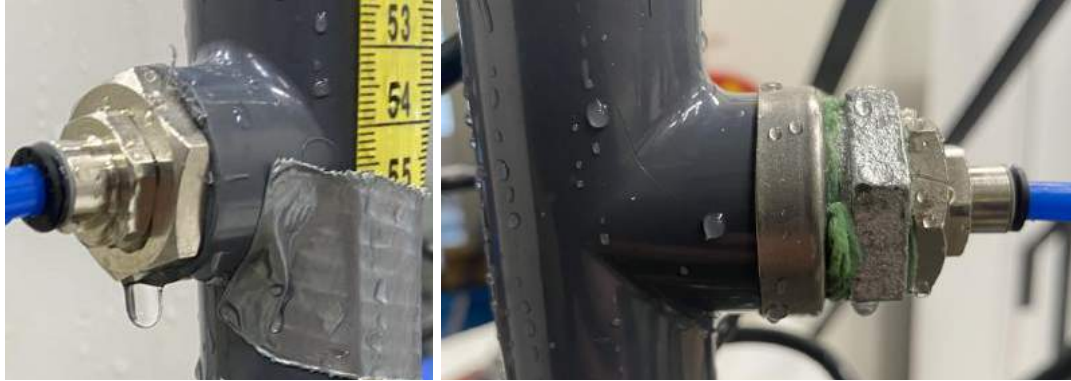
Figures 6.14 and 6.15: The plastic connection (6.13) to the pressure gauge in the water column was replaced by a metallic connection (6.14).
