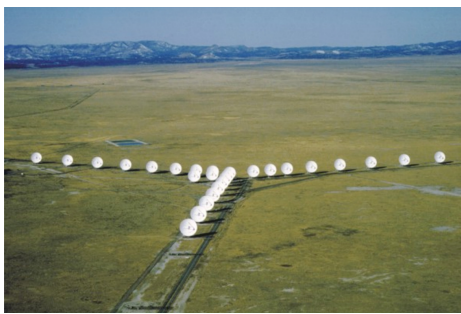
Figure 1: Above view of the Very Large Array in D-configuration. Maximum baselength of each arm is now 1 kilometer. Image from Perley et al. (2011) .
