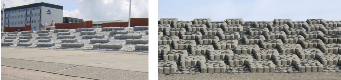
Figure 9: Examples of roughness elements: rib setting (left) and chessboard setting (right). Image adopted from [18].
